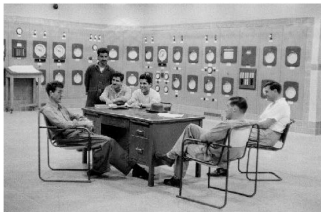
English and Iranian officials during night shift in the control room of the Catalytic Cracker, which breaks crude oil into its various by-products.
